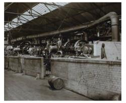
Pelabon steam engines showing the main factory flue. © Guy Pelabon
